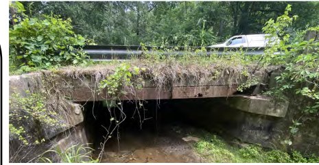
Example of major deterioration of a bridge crossing on Neptune Road.
