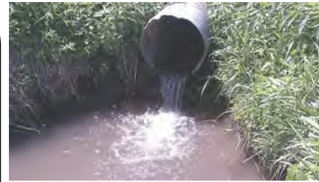
Example of an aquatic barrier due to perching at Kate Ave stream crossing of a trib to the Little La Crosse
