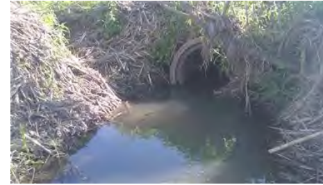
Example of a high flood risk stream crossing (score of 35) at the 1st crossing from Co Hwy J and a trib to the Little La Crosse.
